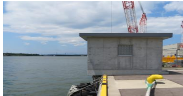
Fig.3 Tide station in Toyama New Port (Fig.1(B))
